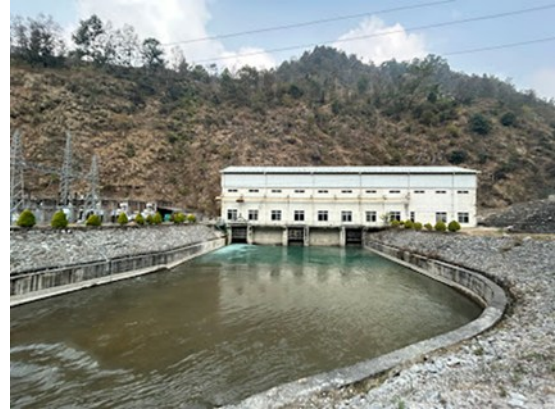
Figure 7: Balephi Hydropower Plant
