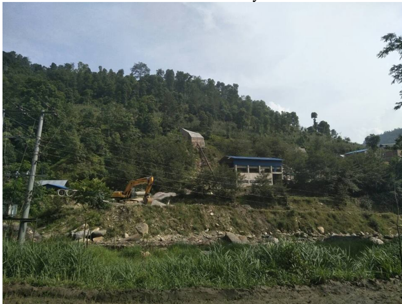
Photo : Gelun Khola Powerhouse
