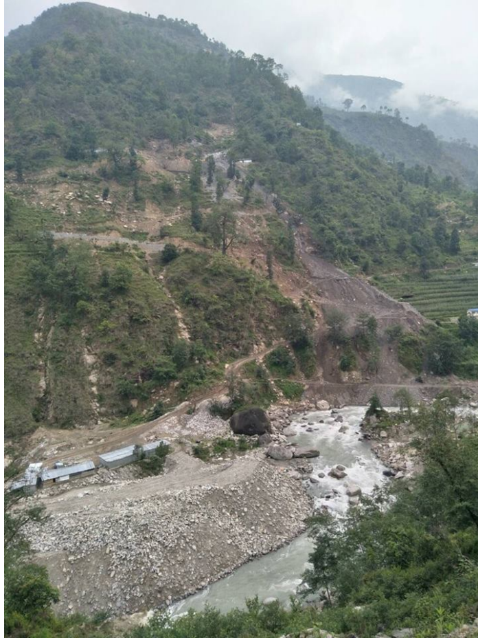
Photo : Hydro Project Tunnel Under Construction in Jugal
