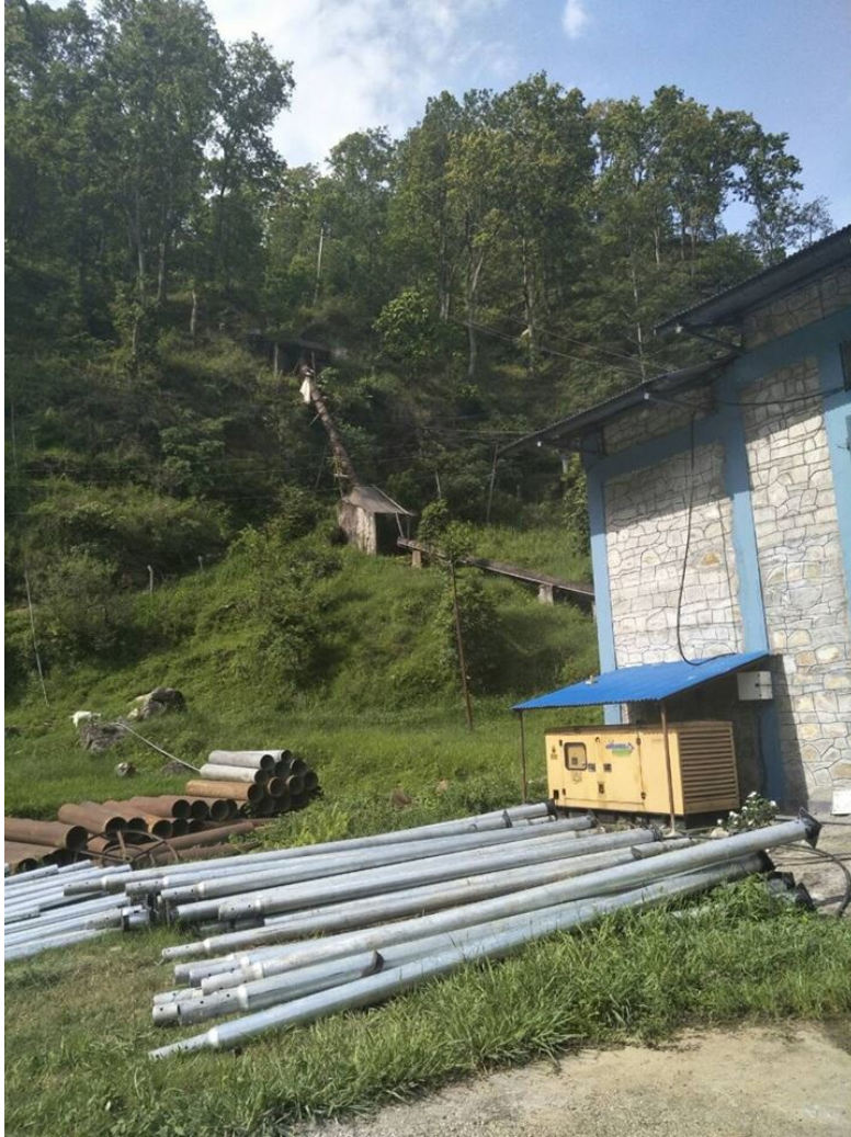
Photo : Baramchi Hydro
